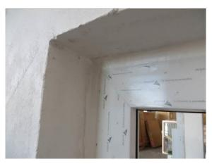
**Photo 3**Corner design of sealing, outside at top
