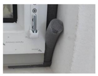
**Photo 2**Detail view, backfilling of sealant joints
